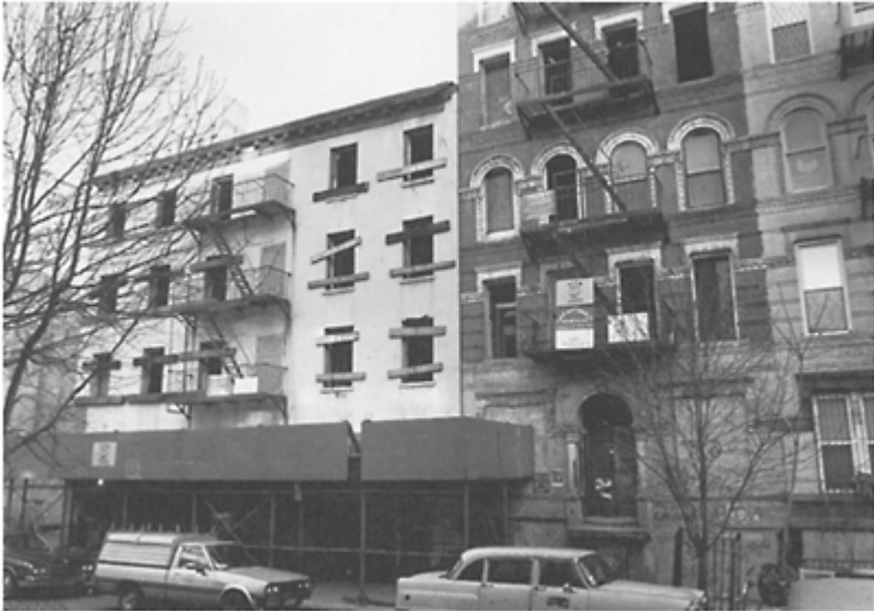
Plate 3.1 Disinvestment in the urban housing stock: an abandoned building and community-based rehabilitation ( The Shadow )
